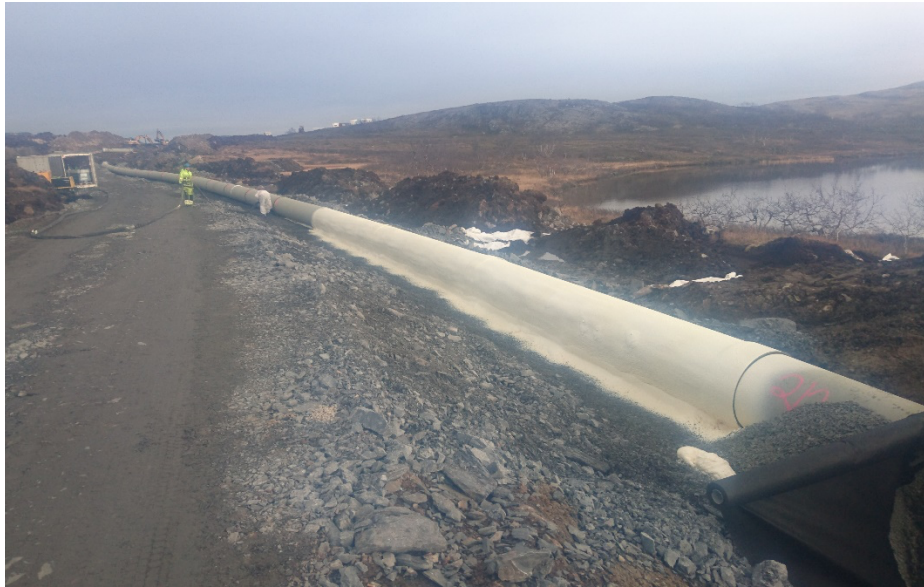
Fig. 1 PU-foam used as backfill
